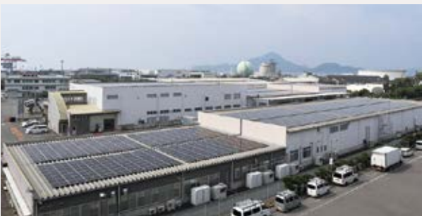
Heart's headquarters factory
