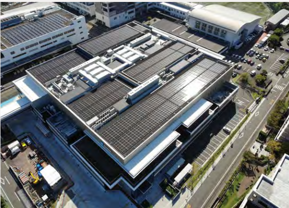
Solar panels installed at the BHCPDII
