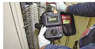
Inspection of electrical equipment at directly operated amusement facility
