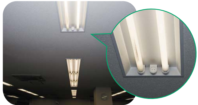
Only two out of three tubes are installed, but the room is bright enough.
