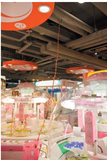
Power cords run along the ceiling
