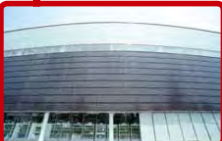
Solar panels installed on exterior walls
